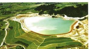
and tailings are disposed of separately to form waste dumps and tailing dams, at Martha the waste rock is used to form engineered earth embankments behind which the tailings are deposited.
